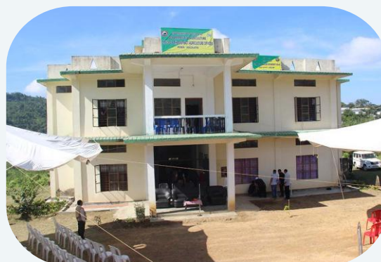
Newly constructed DAO Peren Office
