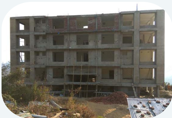
New Directorate building construction in progress
